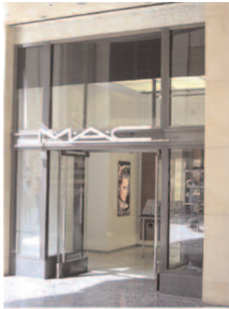
HOLLYWOOD & HIGHLAND ENTRANCE OF KODAK THEATRE
