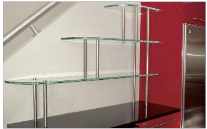
Residential Standoff Project Using 3/4" (19 mm) Custom Standoffs
