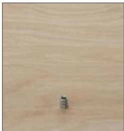
Set Fastener into Surface
