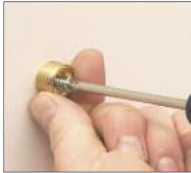
Set Threaded Insert to Wall
