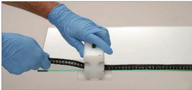
Apply Duralite® to clean glass surface with DSPT1 Applicator or by hand.
