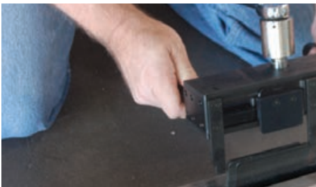
Place Installation/Removal Tool into position onto the Tapers and push them down into the Base Shoe.
