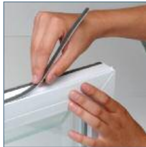
Remove old Pile from frame
