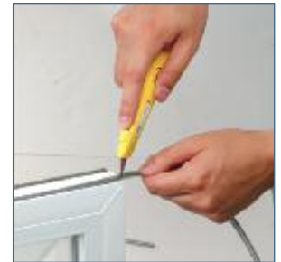
Cut to length with knife or scissors
